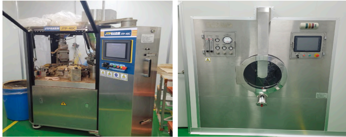
Capsule Room Coating Room
